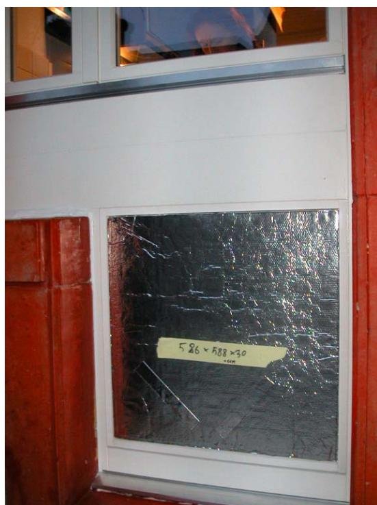
Figure 36: Window element with tight-fitting VIP
