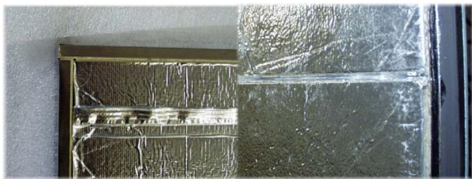
Figure 57: Gaps and edges of VIP in the elements
