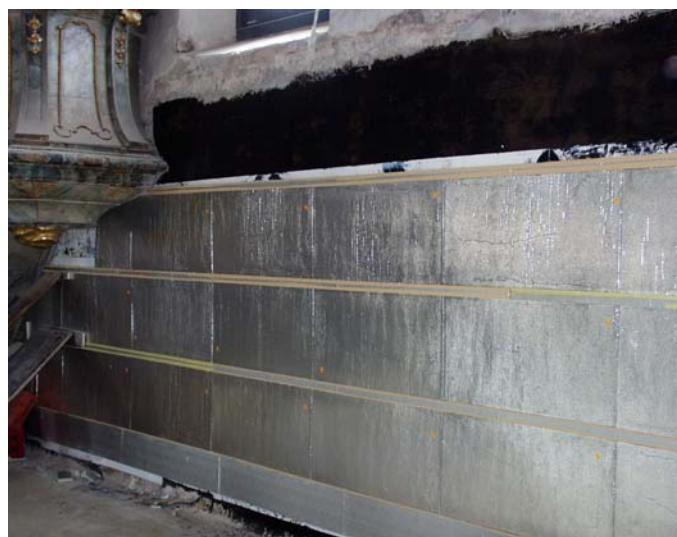
Figure 52: Left: Installation of the VIP with dispersion based mortar onto the polysterene boards. The horizontal strips of polyurethane can be seen as well as the vertical strips of dispersion based mortar.
