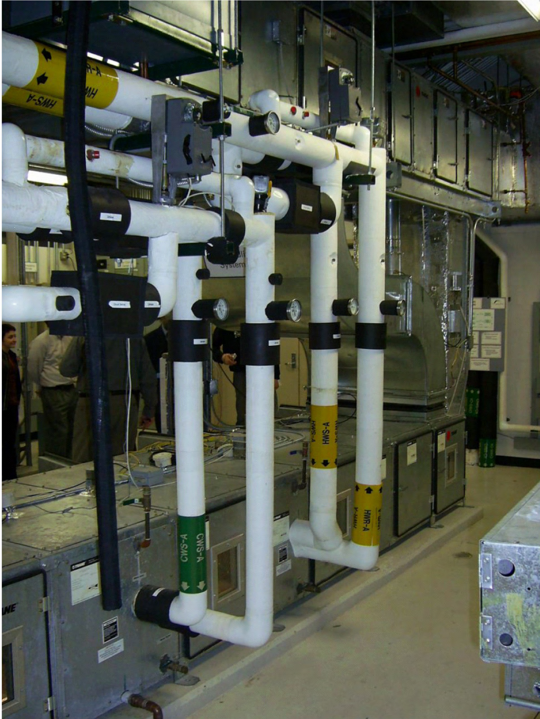
Figure 2-3 Outside view of the AHU
