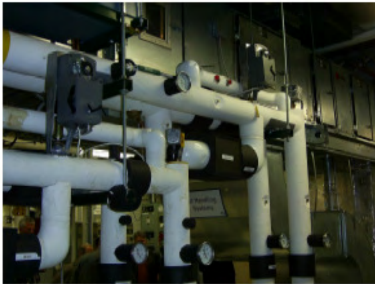
Figure 5-2 Hydraulic connections with mixing valves (heating and cooling coil)
