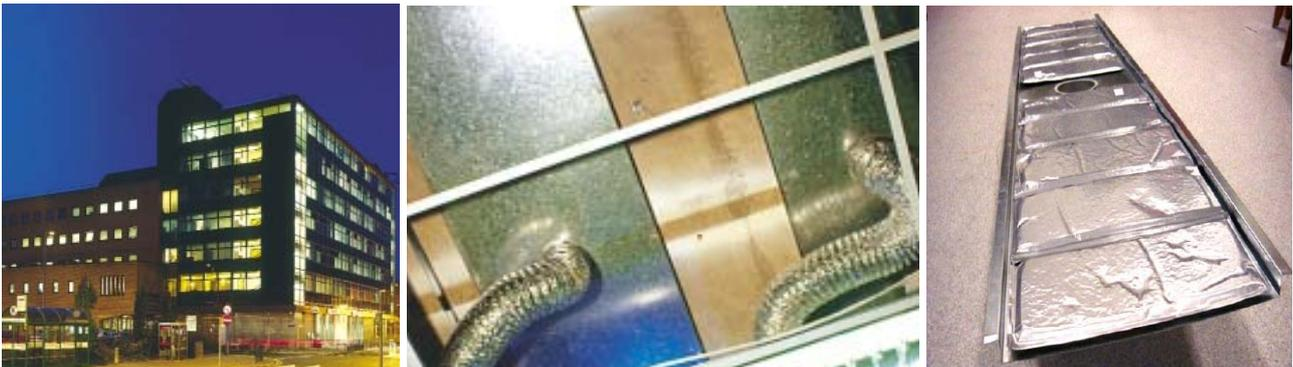
Figure 7.20 – Picture of the “Stevenage Borough Council “ building – Construction details of the PCM based ceiling (Cooldeck technology).
