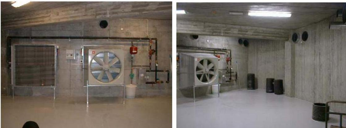
**Figure 6.19 - The air distribution room, showing the preheat unit (left) and fan, as well as the plastic subterranean ducts leading to the various rooms [Schild (2002)].**
