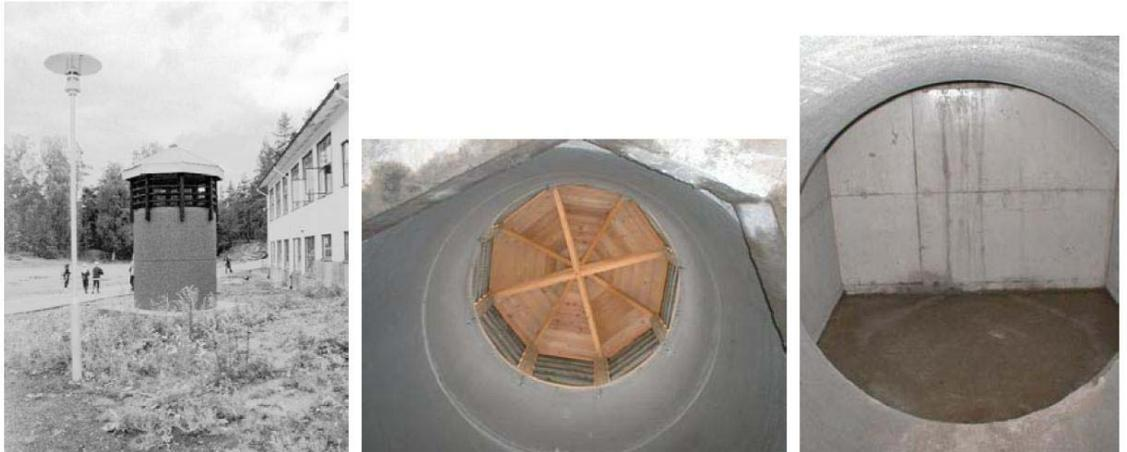
**Figure 6.18 - Jaer School air intake tower (Left: outside, Middle: inside looking up, Right: inside horizontally into base of the tower from the horizontal ETAHE duct.) [Schild (2002)].**
