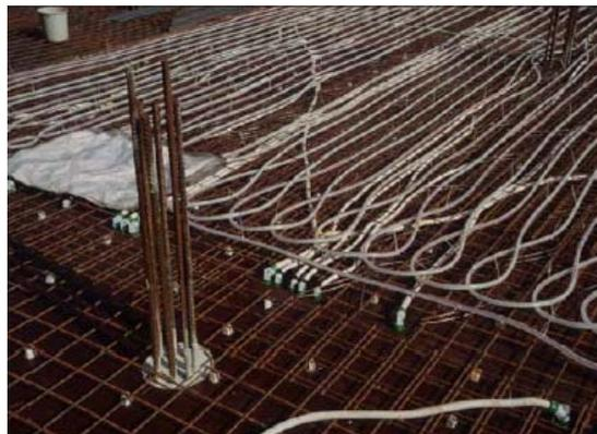
**Figure 5.9 - Concrete lying on the reinforcement grid with attached pipes [Hauser et al.( 2005)].**
