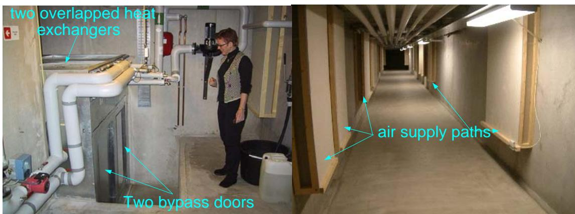
**Figure 6.15 - Air distribution duct of Mediå school (Left photo shows heat exchangers and "summer" doors. Right photo shows the supply air paths) [Tjelflaat (2002a)].**
