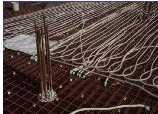
Figure 3-24 Concrete lying on the reinforcement grid with attached pipes
