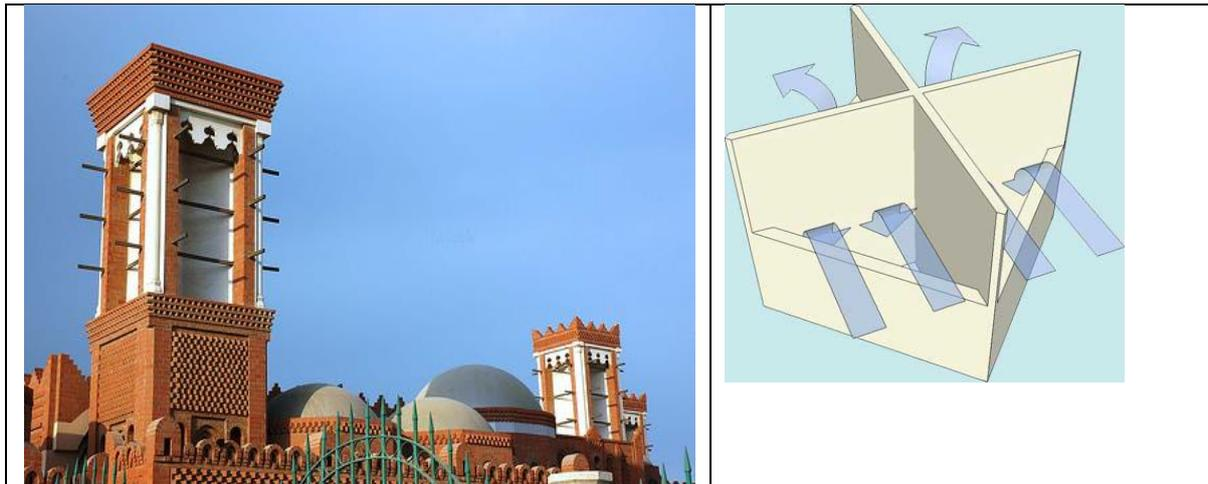
Figure 5.29. Traditional windcatcher at Qatar and sketch of functional principle Figure 5.28. Traditional windcatcher at Qatar and sketch of the functional principle of a square bidirectional windcatcher with four sections. Sources: [www.trekearth.com](http://www.trekearth.com) and <http://catnaps.org/islamic/gulfarch4.html> (29.07.2014)
