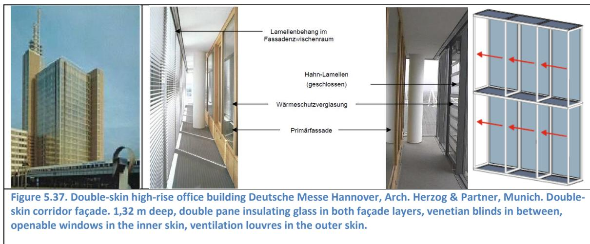
Figure 5.37. Double-skin high-rise office building Deutsche Messe Hannover, Arch. Herzog & Partner, Munich. Double-skin corridor façade. 1,32 m deep, double pane insulating glass in both façade layers, venetian blinds in between, openable windows in the inner skin, ventilation louvres in the outer skin.
