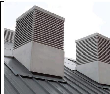
Figure 5.25. Prefab Airstract Ventilator utilizing Venturi effect. Passivent, GB
