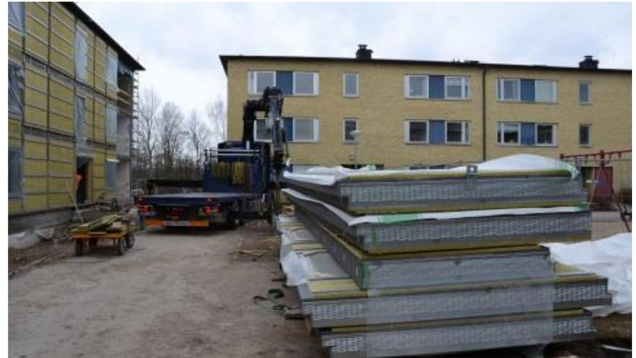
*Prefabricated facade elements for the next phase of renovation.*
