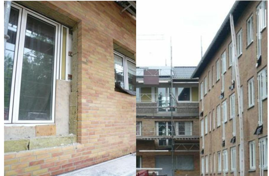
*190 mm insulation plus exterior solid standard bricks. Energy windows – aluminium – wood, 3-layer energy glass. In the panel walls: 285 mm insulation plus exterior solid standard bricks.*
