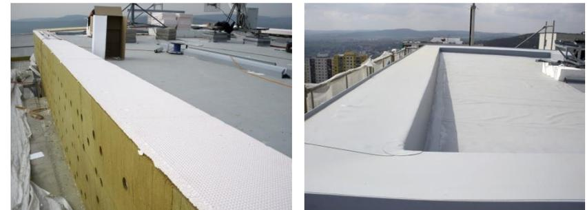
The attic during the renovation - installation of additional thermal insulation over the attic to reduce the thermal bridge (left) and a view of the new waterproofing/covering layer made of mPVC sheets (right). Precise design and construction of structural details are crucial for proper function of any energy efficient building. [1]
