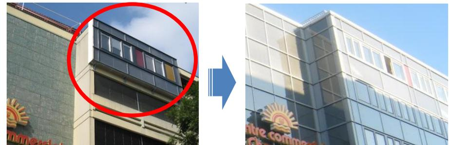
*Pre-fabricated solar facade system from gap-solution*
