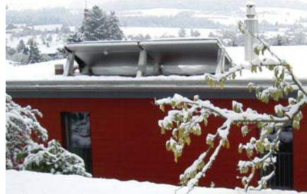
Solar thermal collectors and weather sensor on the roof
