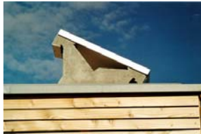
Photovoltaics installation on the roof
