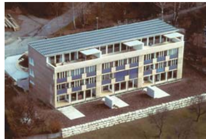
PV installation on the roof
