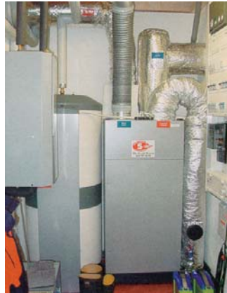
Plant room: Expansion tank of the solar collectors, boiler, compact ventilation unit with integrated mini-heatpump and controller for the solar system.
