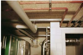
Special (Hilti) construction from wall to wall without penetration of insulation
