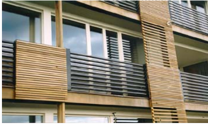
South facade with vacuum collectors as balcony railing
