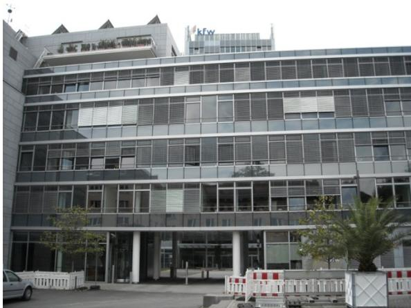
Figure 2-38: Two-part sun protection enables glare-free use of daylight
