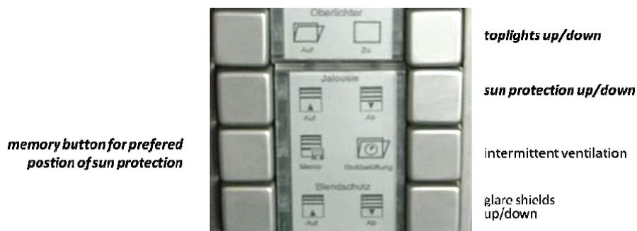
*Figure 2-41: Control device and its functions*
