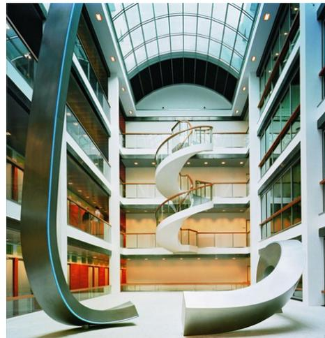
Figure 2-37: The atrium lights the traffic areas and enables natural ventilation
