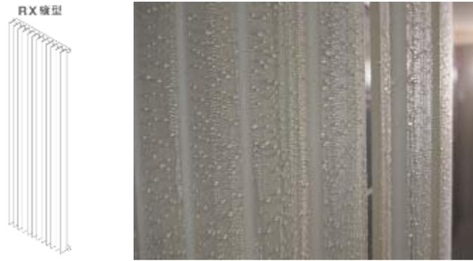
Fig. 4-30 Example of dehumidifying chilled radiators
