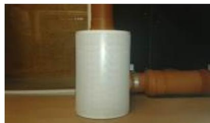
Fig. C-2 Wall displacement diffuser QL – WH – R0.
