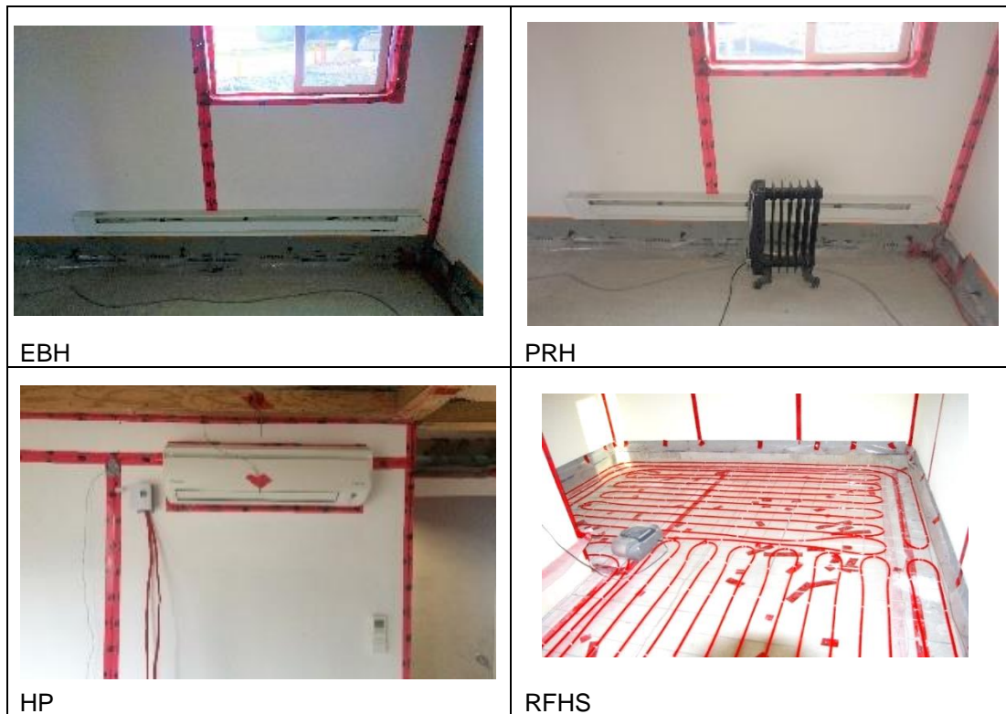
Figure 40 - Heating systems considered in the study.
