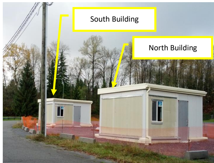
Figure 51 - Two test building facilities used for the experimental study.
