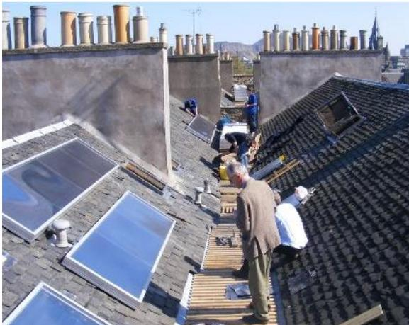
Figure 6: Installation of the solar thermal units, © HES
