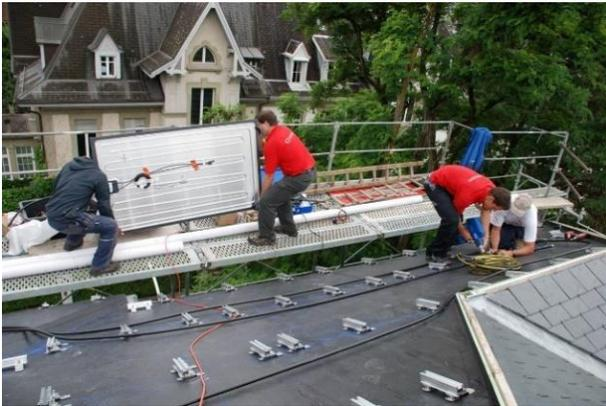
Figure 99: Single family House, Bern. Installation of PVT+PV panels, © M. Hutterli
