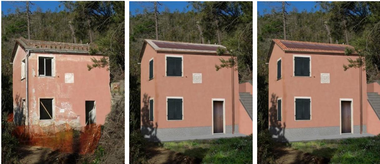
Figure 128: Simulation of a new coloured PV roof (almost integral) on slate or on tiles. A) the current state, b) the new roof inserted on slates, c) the new roof inserted on tiles (FAI).
