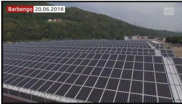
*Figure 122: The plant in Barbengo, an example recently built: 7'000 thousand square meters of surface covered with panels will provide energy to over 200 families. An initiative project of the Companies industrialists of Lugano, who support the work, in return from this roof will yield 1,000 megawatt hours per year, that is. energy for 220 families, as part of the "Sun" project for all", © RSI 2018*
