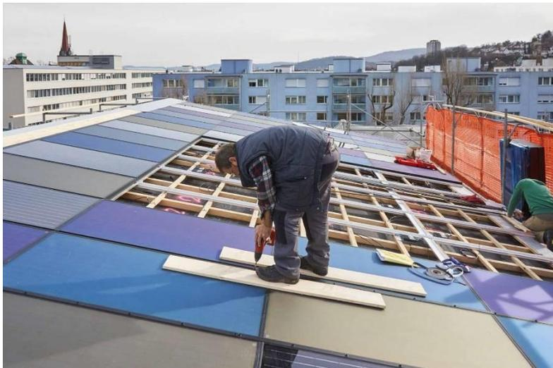
Figure 139: Installation of PV and BIPV modules on the Roof, © Martin Zeller
