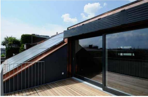
*Figure 16: Roof with solar thermal and PV, Viridén + Partner AG Architects, © Nina Mann*
