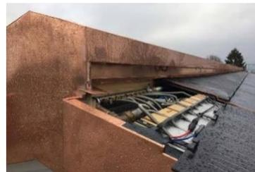
Figure 30: PVT panels, new roof. © D. Studer, Studer Architekten
