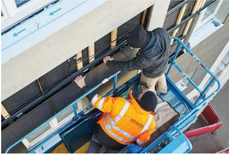
Figure 138: Installation of PV modules on back rails, . Picture: © Martin Zeller
