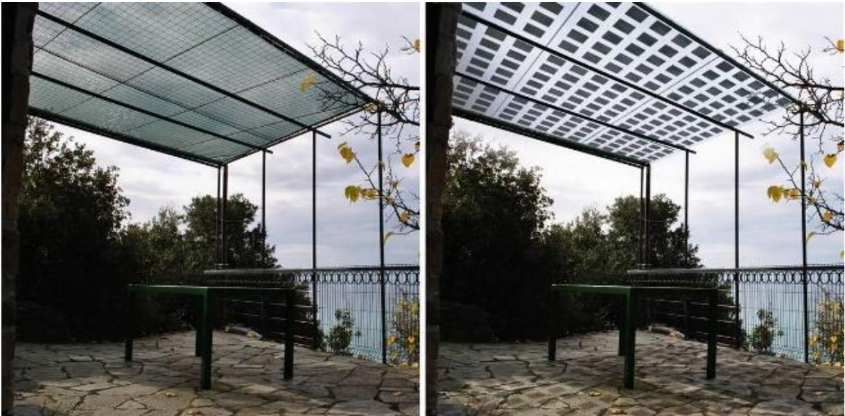
Figure 125: Monestiroli, photo-simulation of a compatible intervention. On the left, current state, on the right, the use of transparent PV cells
