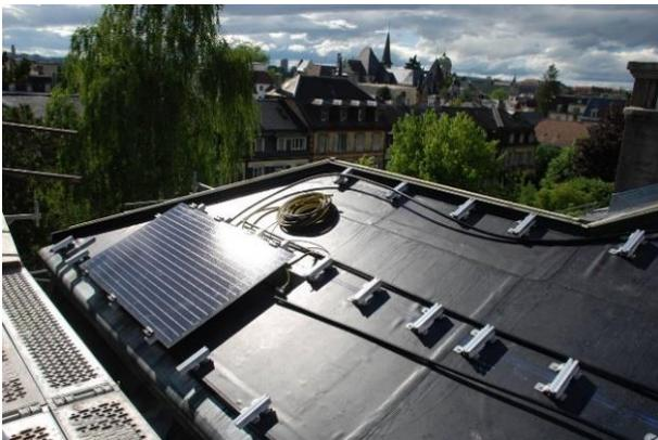
Figure 100: Single family House, Bern. Installation of PVT+PV panels, © M. Hutterli
