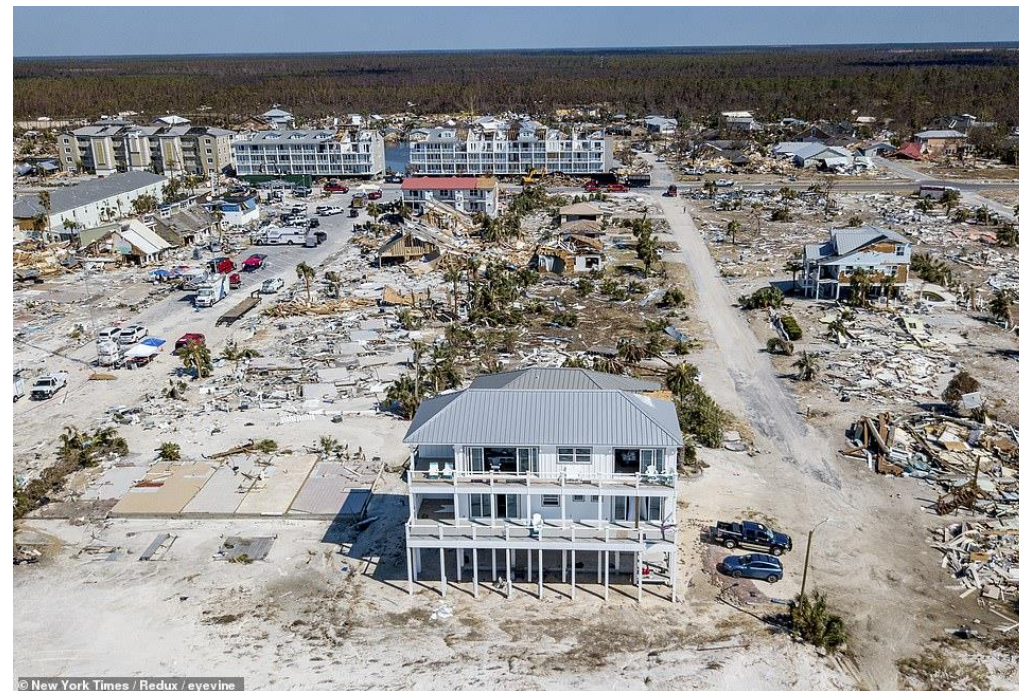
Image of Mexico Beach, Florida home following Hurricane Michael
