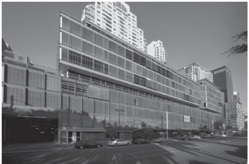
The new Bovis Lend Lease HQ at 30 The Bond, Australia's first commercial building to commit to a five star energy rating from SEDA (The Sustainable Energy Development Authority)
