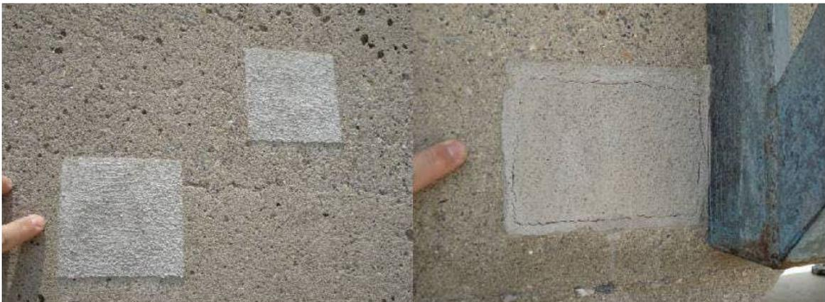
**Figure 4-12. Typical repairs using a cementitious material. The patch material has a rough appearance and failed within months of installation.**
