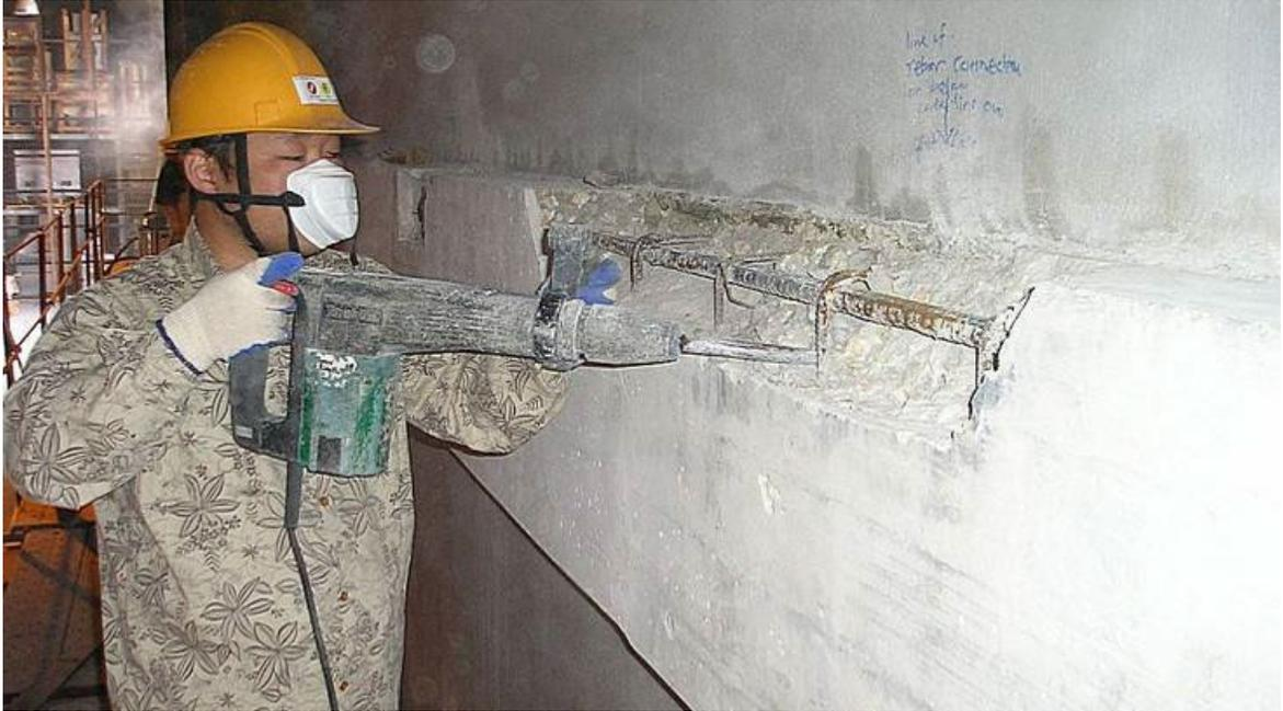
**Figure B-4. Concrete repair.**
