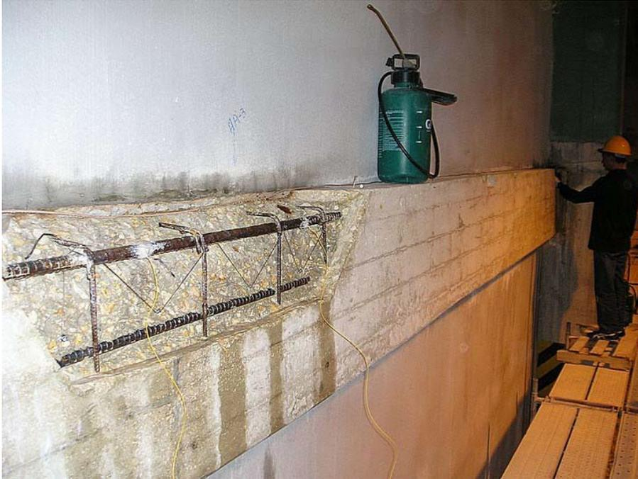
**Figure B-7. Electrical connections to the rebar were made to facilitate future testing.**
