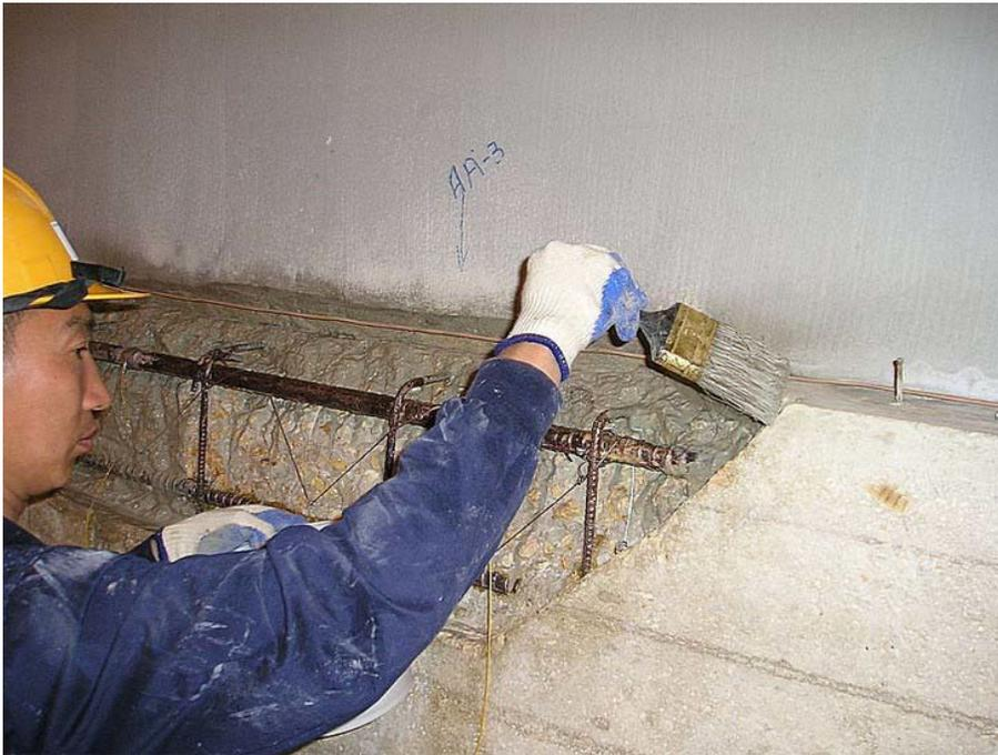
**Figure B-10. Concrete repairs were placed and finished in accordance with generally accepted construction practices in all locations on the ring girder side 1 (Surtreat system).**
