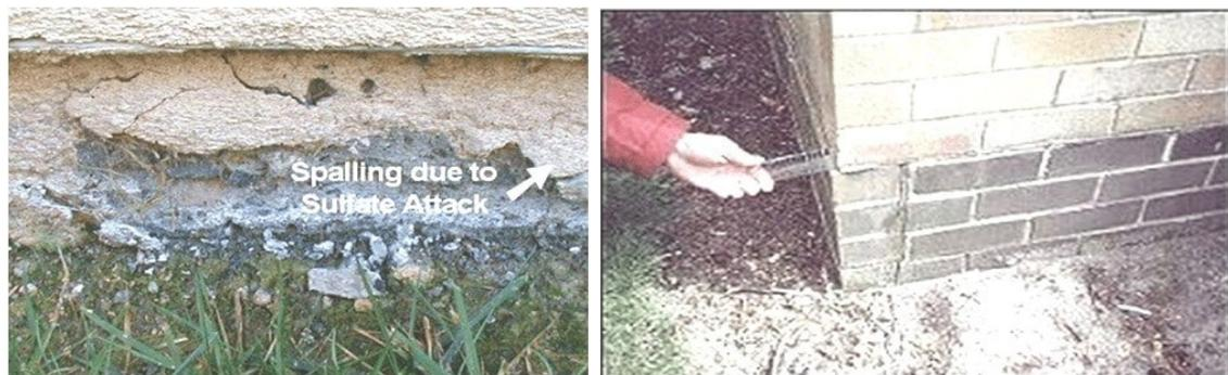
**Figure 1-12. Spalling due to a sulfate attack.**
