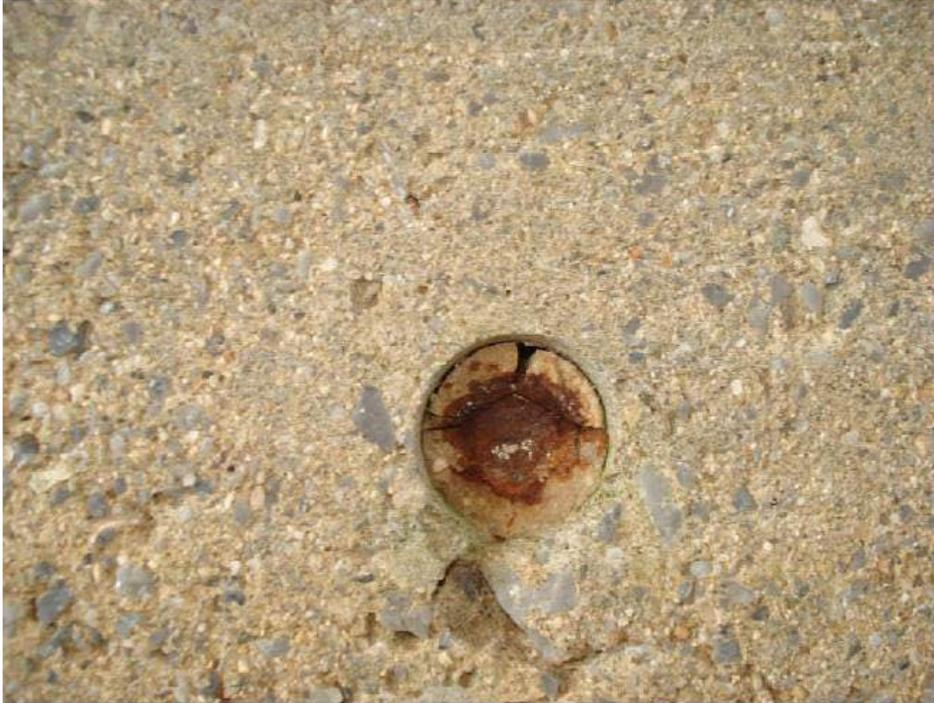
**Figure 4-13.** Shows a typical corroded steel rebar that has delaminated from the concrete.
