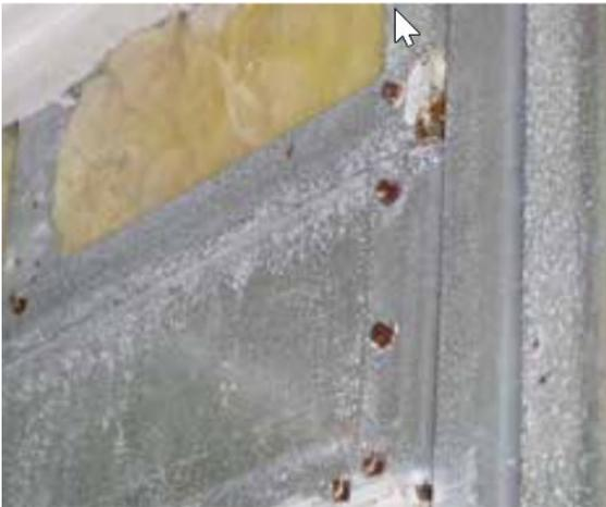
**Figure 1-4. Example of corroded fasteners.**
