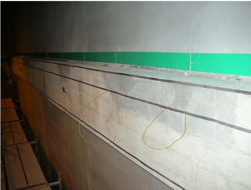
Figure B-15. Appearance of the Ring Girder Side 2 immediately after application of the LGC.
