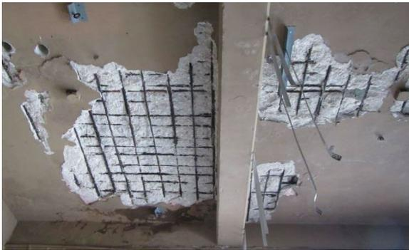
**Figure 1-7. Common spalling of concrete.**
