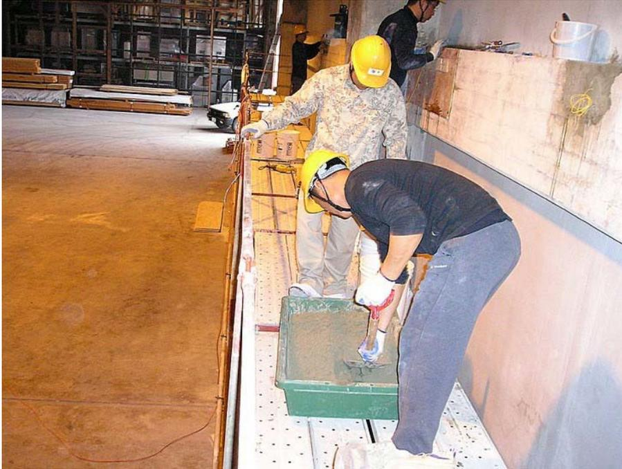
**Figure B-9. Concrete repairs were made following corrosion inhibitor system application to the demolished delamination areas.**
