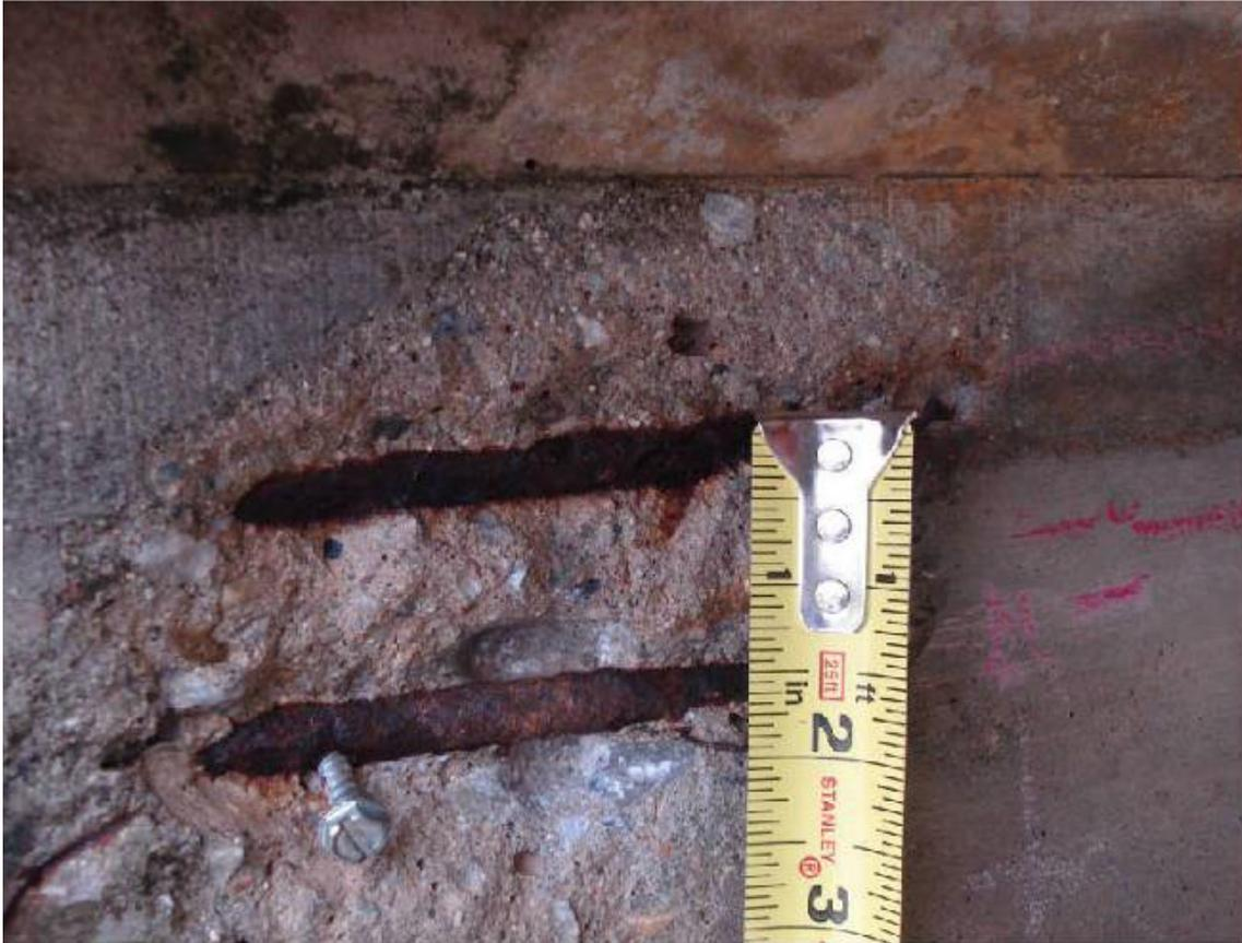
**Figure 4-11. Exposed rebar on culvert.**
