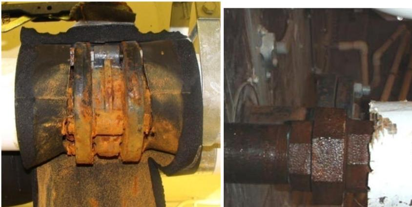
**Figure 1-15. Corroded union joints on piping in a mechanical room.**
