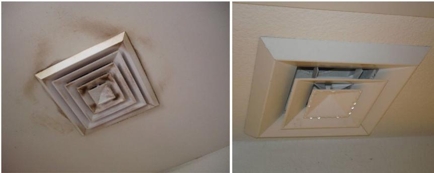
Figure 5-18. Condensation on ceilings and diffusers.
