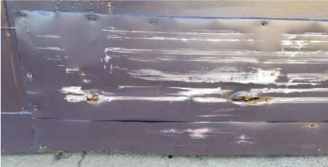
**Figure 1-6. Door damage by machinery impact.**
