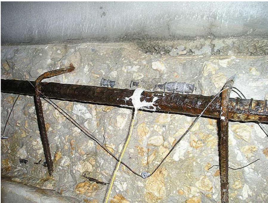
**Figure B-8. Concrete was mixed from local masonry with polymer added for improved strength and durability.**
